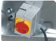
Fan fitted with INT series safety switch
